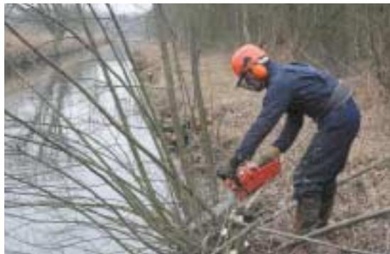
Scrub clearance and promotion of reed growth are effective in providing natural banks, which have the ability to absorb and dissipate wave energy thus reducing erosive forces.
