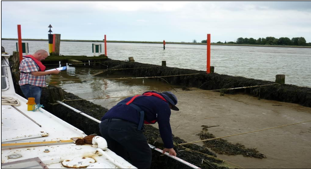
Photo: New steel cable ties and markers seen during recent survey
