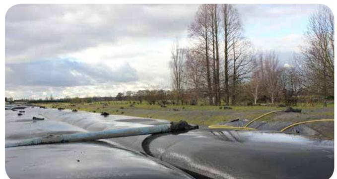
*Through the large tube in the middle the sediment is brought in geotextile tubes. The water leaves the tube through the "pores" in the geotextile*
