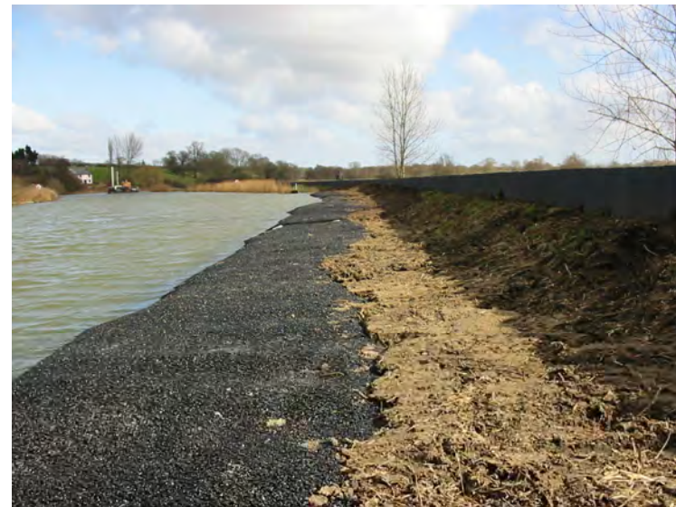
PHOTOGRAPH OF ROND IMMEDIATELY AFTER INSTALLING EROSION PROTECTION
