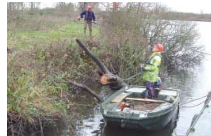
Tree clearance at Train Reach on the River Yare
