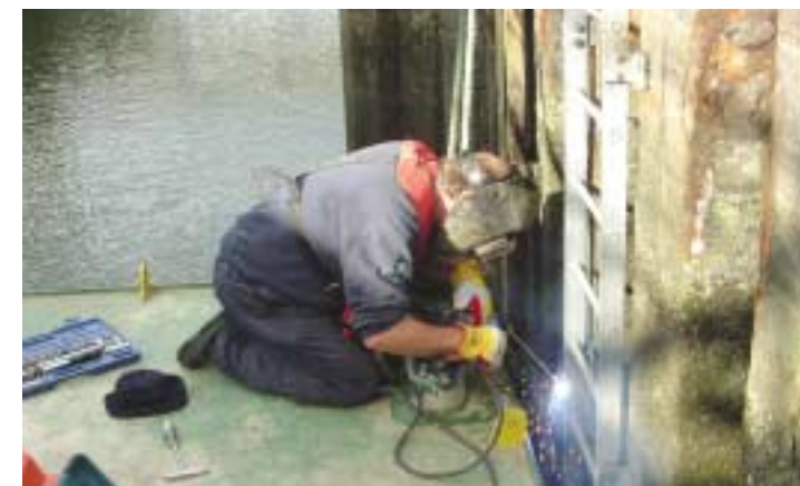
Installing a ladder at Mutford Lock
