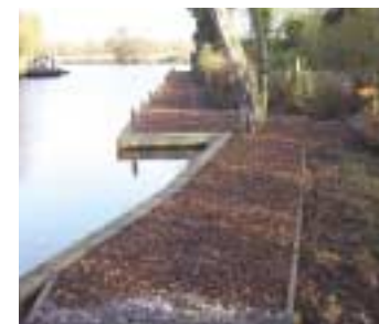
Cockshoot Dyke mooring before and after refurbishment
