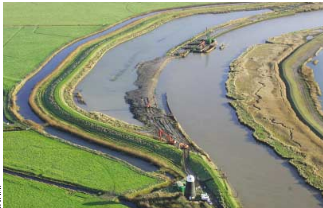
Set back flood defences at Seven Mile House, River Yare
