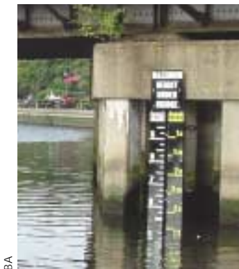
New gauge board at Thorpe Viaduct
