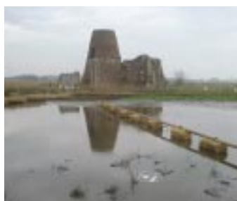
Mudpumping at St Benet's Abbey
