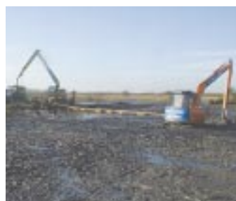
Disposal of dredgings at St Benet's for land raising
