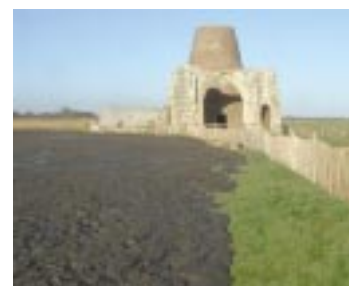
Disposal of dredgings at St Benet's for land raising
