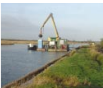
Dredging at Thurne Mouth
