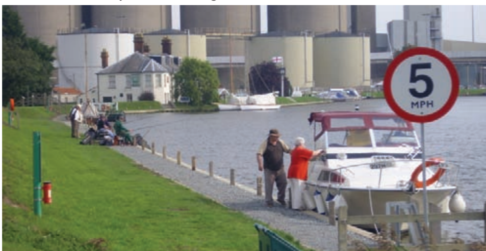
The refurbished Cantley 24 hour moorings
