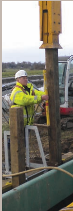
Driving in piling to protect safety ladders
