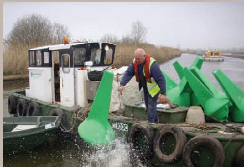
Placing channel markers
