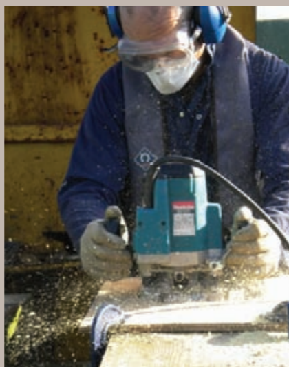
Preparing timber for quay heading
