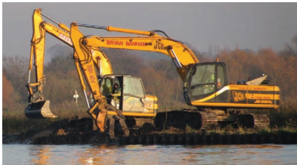
Removing hazardous piling at Upton Marshes
