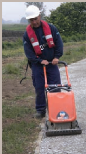
Compacting a path
