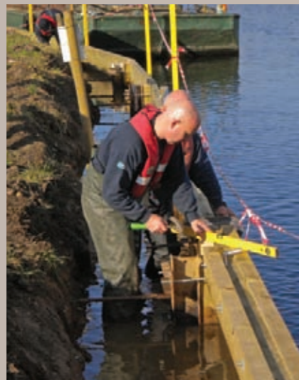
Installing new quay heading timbers
