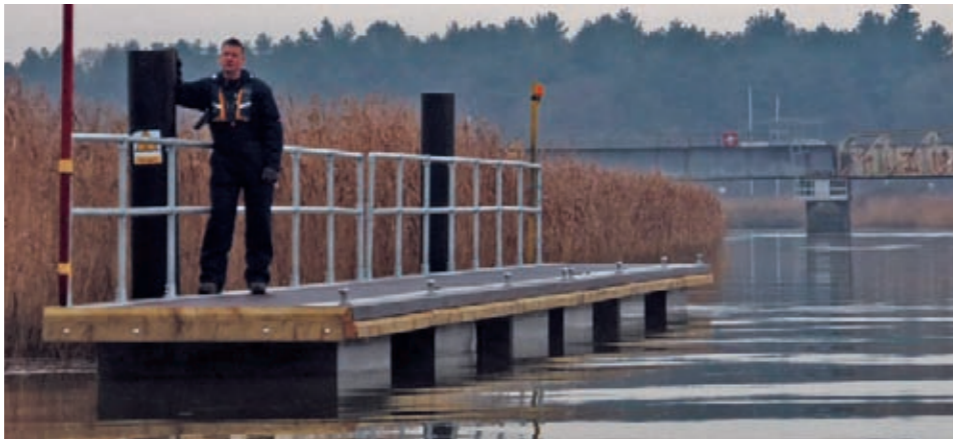
New lay-by pontoon at Somerleyton Bridge
