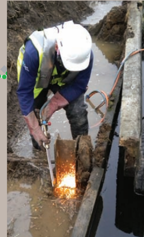
Cutting steel work
