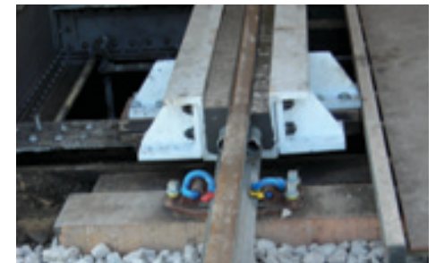
Bearing plug out - the main swing bearing sees the light of day for possibly the first time in 100 years
