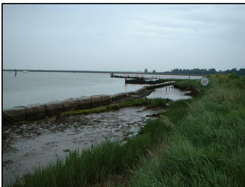
Compartment 35 – Haddiscoe Island. Gabions installed awaiting dredgings behind.
