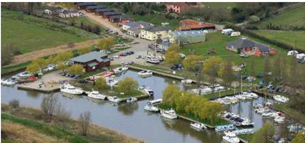
Aerial View of Waveney River Centre (from website)
