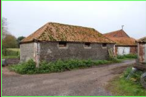
Fig 22, Cobble walled farm building at Mill Farm
