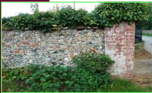
Fig 23, Cobble and brick rubble wall, Floral Loke c1820
