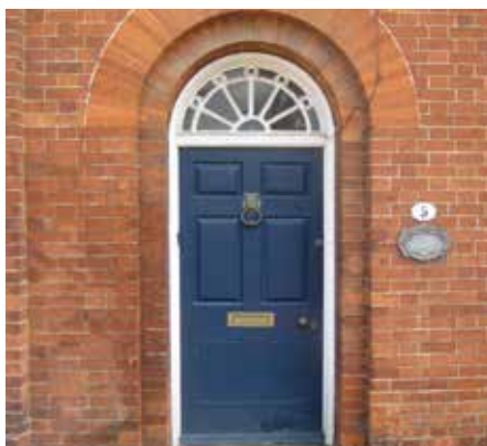
Fine gauged brick arch with decorative fanlight, Beccles Rd
