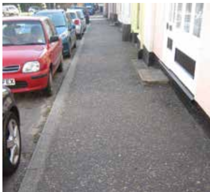
Tarmacadam and chippings with granite kerbs in The High Street.
