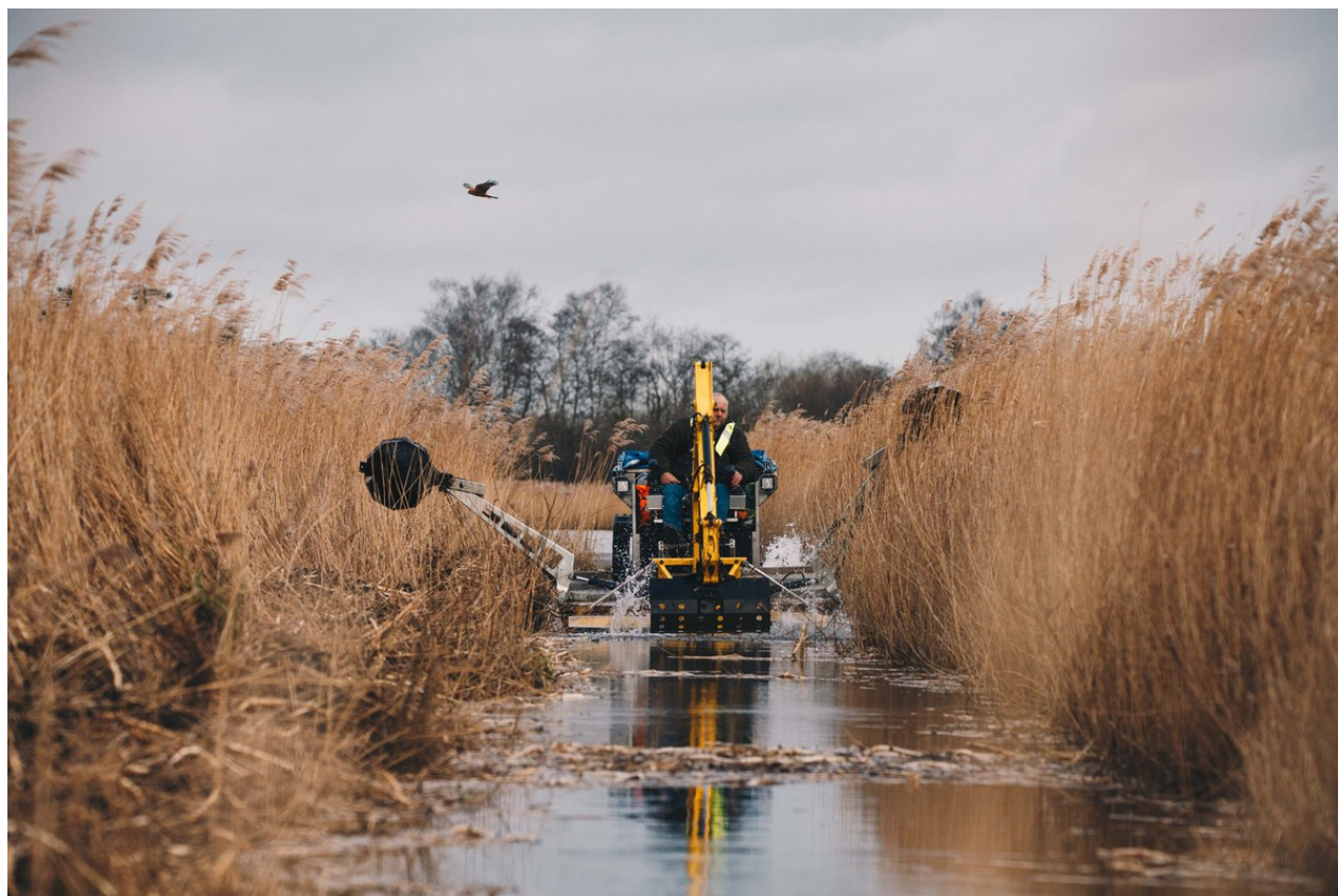
Photo: Amphibious digger excavating lost ditches in reed beds © Broads Authority
