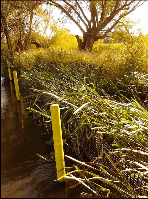
Photo 4: Nicospan erosion protection structure planted with bur-reed.
