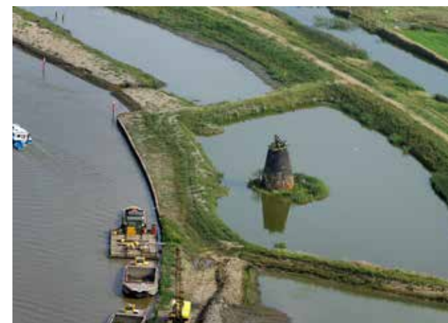
Six Mile House surrounded by water. Efforts are underway to conserve it for the future by infilling the lagoon within which it sits with dredged material. Mike Page
