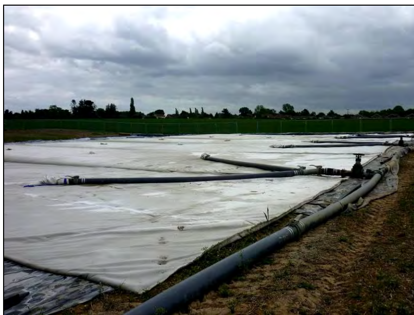
Photo 2: Geotextile bags starting to be filled at Upton
