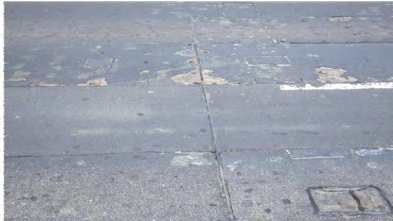
Typical Anti Slip Surface Lose
