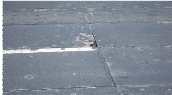
Broken Corner to Deck Board
