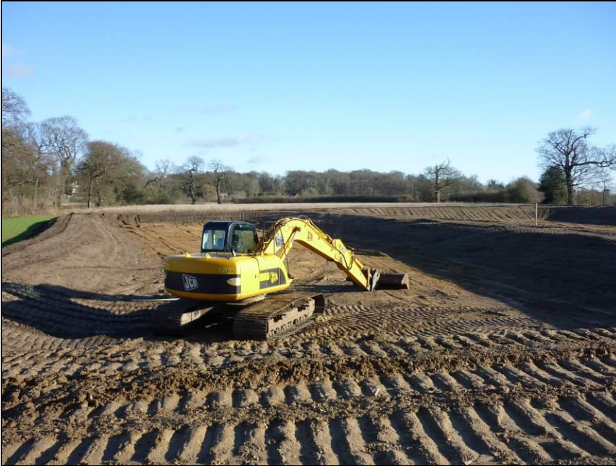
Photo 3: Constructing settlement lagoons near Coltishall
