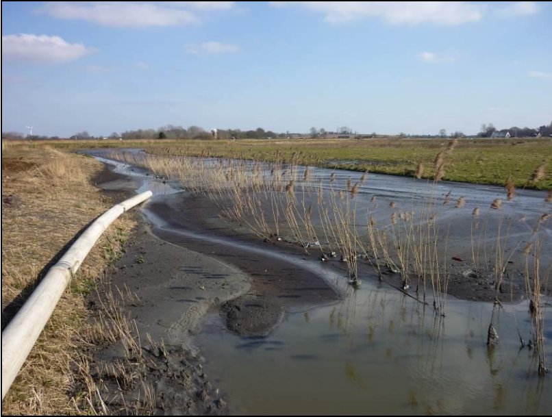
Photo 5: sediment pumped from Heigham Sound filling former soke dyke.
