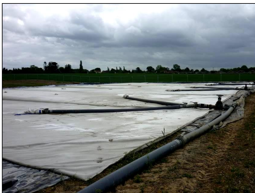
Photo 2: Geotextile bags starting to be filled at Upton
