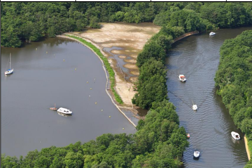
Photo 8: Newly restored reed swamp area retained by geotextile tube at Salhouse Broad.
