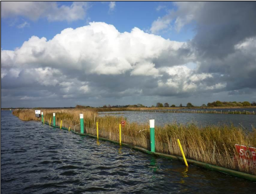
Photo 7: View of the perimeter baskets from the water with reed beginning to establish.
