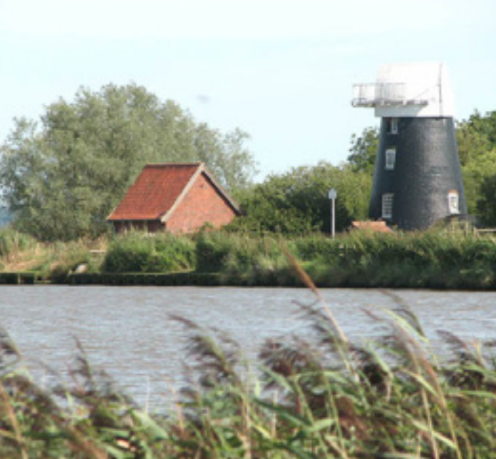
▲ Norton Drainage Mill (now a holiday let) with the internal drainage board pump house how now been demolished. Image by Evelyn Simak - geograph.org.uk
