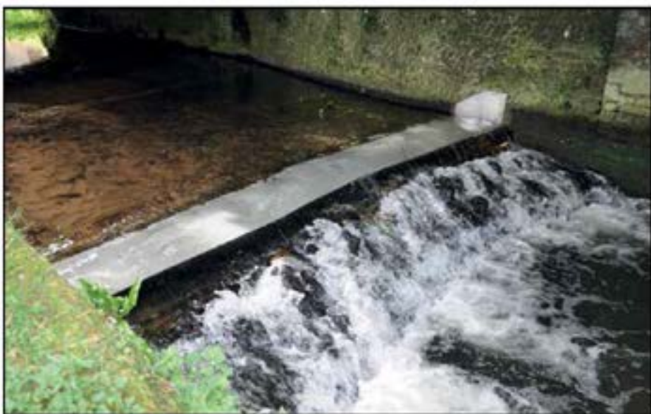
From the top: 1. Concrete topped weir with the river flow reduced. 2. Assembly and fixing of overhanging barrier and side support components. 3. Signal crayfish barrier in place and restored river flow.
