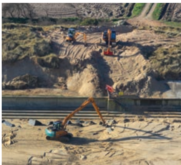
Waxham, Norfolk: Recharging the beach replaces sand and shingle lost to erosion
