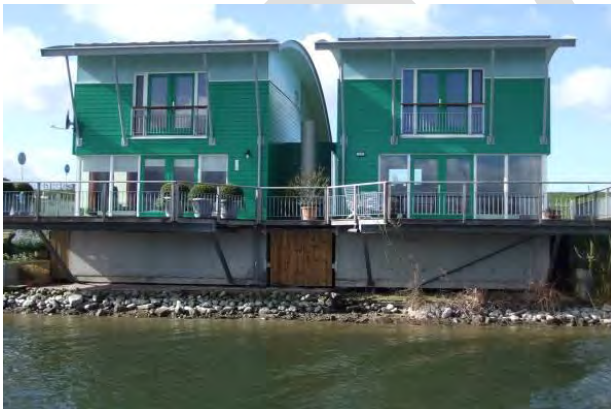
A house on dry land in Holland, which floats if waters swell.
