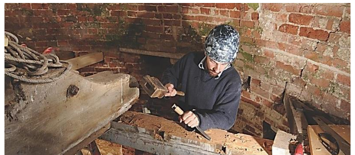
Photo: Millwright repairing floor joists
