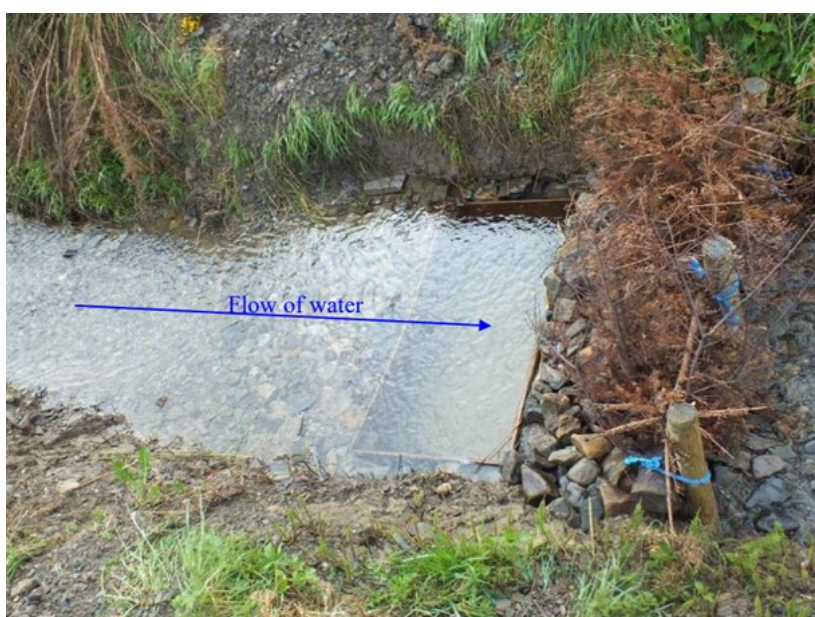
Figure 3.1 Silt trap installed in a stream (Source: IRD Duhallow, 2015)
