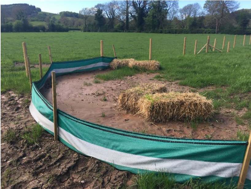
Figure 3.2 Silt fencing installed on agricultural fields (Source: HY-TEX, 2022)
