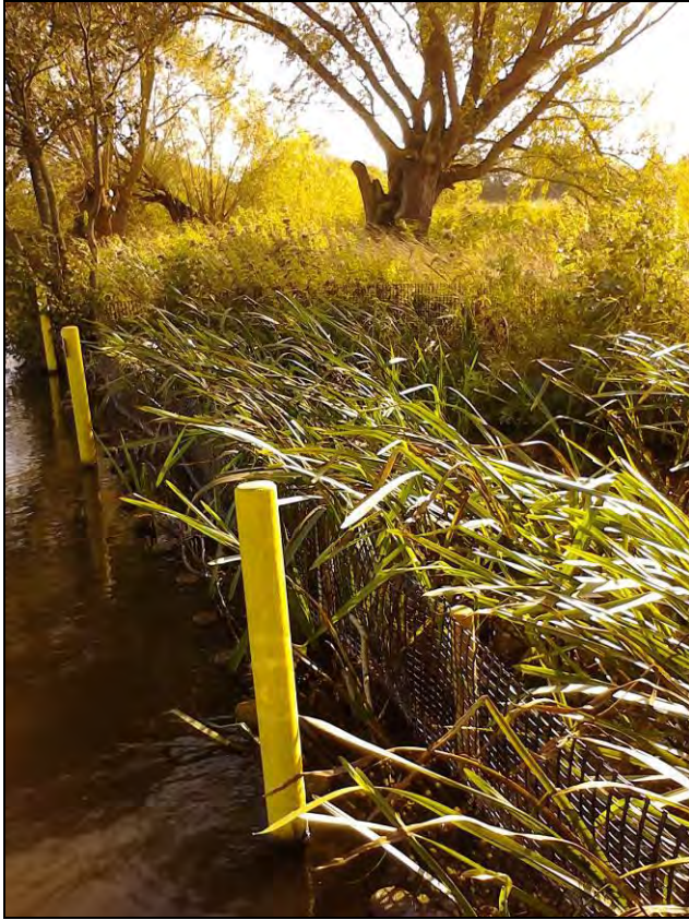
Photo 4: Nicospan erosion protection structure planted with bur-reed.
