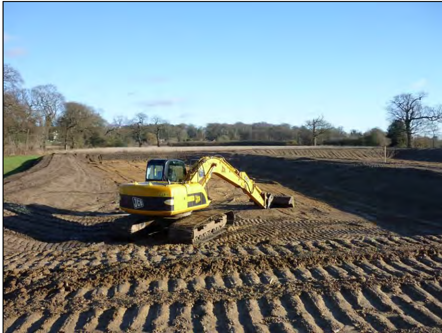
Photo 3: Constructing settlement lagoons near Coltishall
