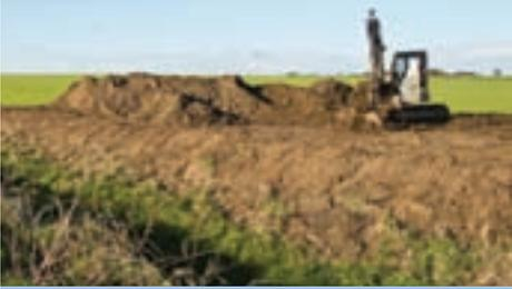
*Constructing an earth bund in an arable field to retain topsoil following heavy rainfall.*
