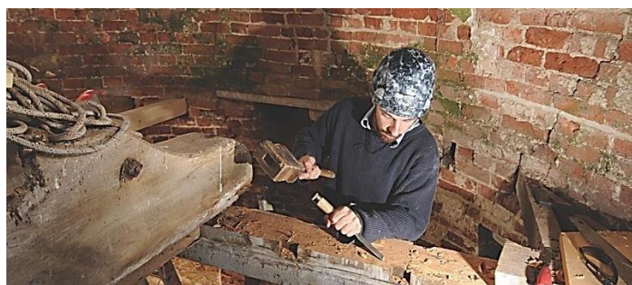
Photo: Millwright repairing floor joists
