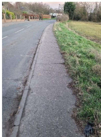
Example of the narrow footway on Waters Lane
