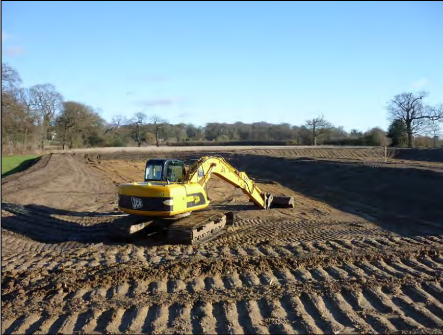
Photo 3: Constructing settlement lagoons near Coltishall
