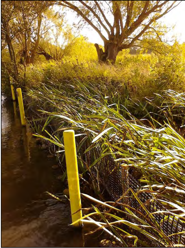
Photo 4: Nicospan erosion protection structure planted with bur-reed.
