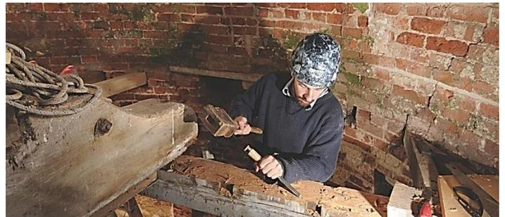
Photo: Millwright repairing floor joists
