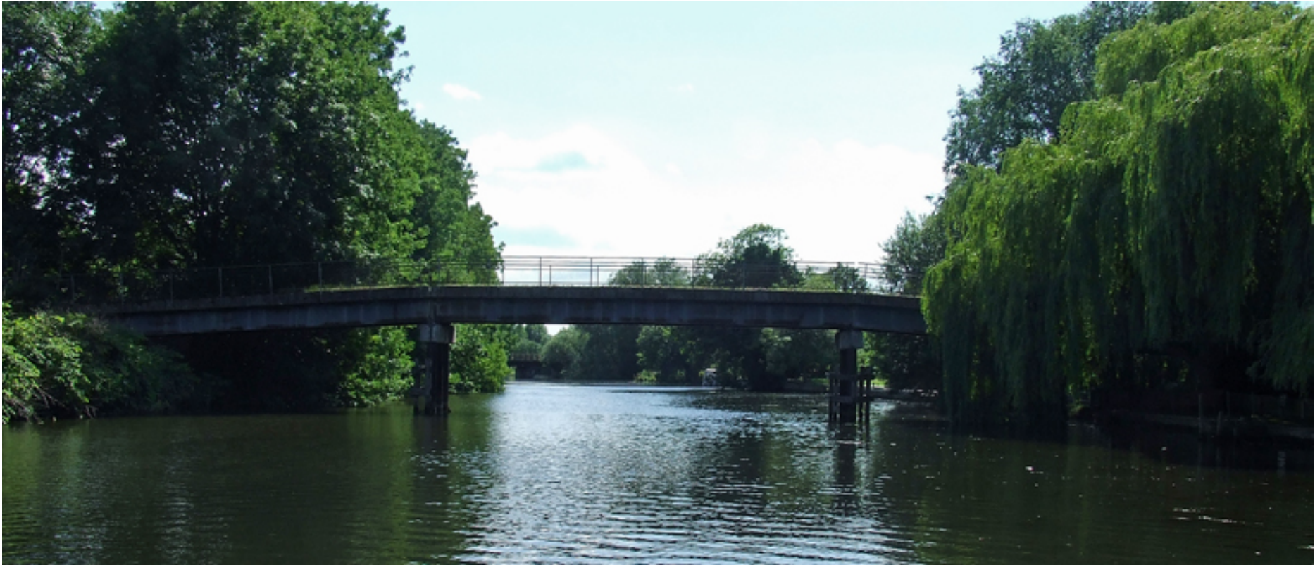
Thorpe Island Bridge
