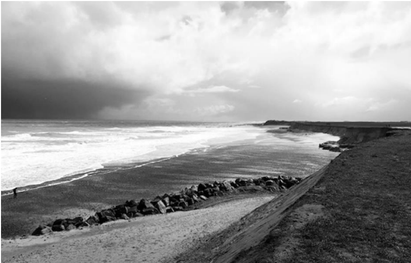
Sea defences/rock berm at Happisburgh with cliff erosion shown
