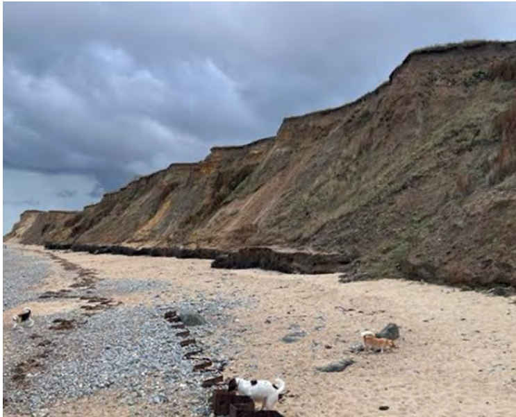
Eroded cliffs at East Runton
