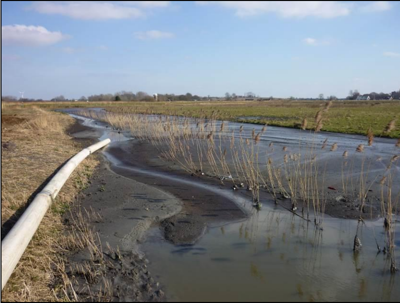
Photo 5: sediment pumped from Heigham Sound filling former soak dyke.
