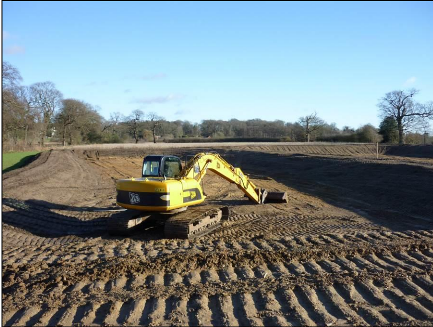
Photo 3: Constructing settlement lagoons near Coltishall
