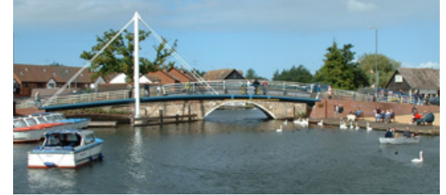
▲ The medieval bridge at Wroxham/ Hoveton, which is the only vehicular river crossing in the locality, restricts the size of boats that are able to travel upstream due to the low arches of the bridge. Image by Keith Evans – geograph.org.uk
