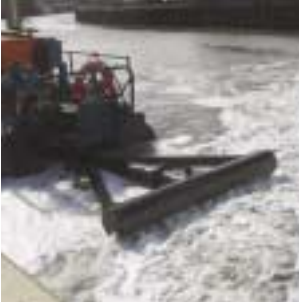
Water injection dredging
