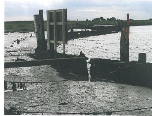
② BROKEN WALING & SLACK TENSION WIRES
