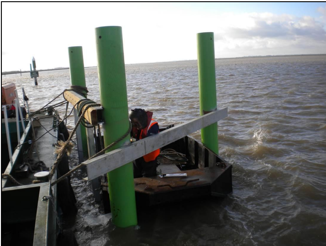
Photo 3: New de-masting dolphin during construction
