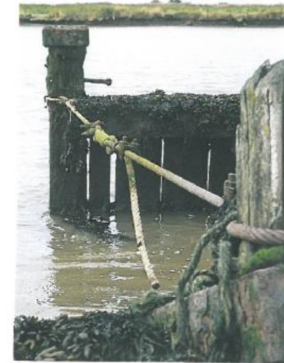
③ TENSION WIRE STILL EFFECTIVE (ADJACENT TO MISSING PILING)
