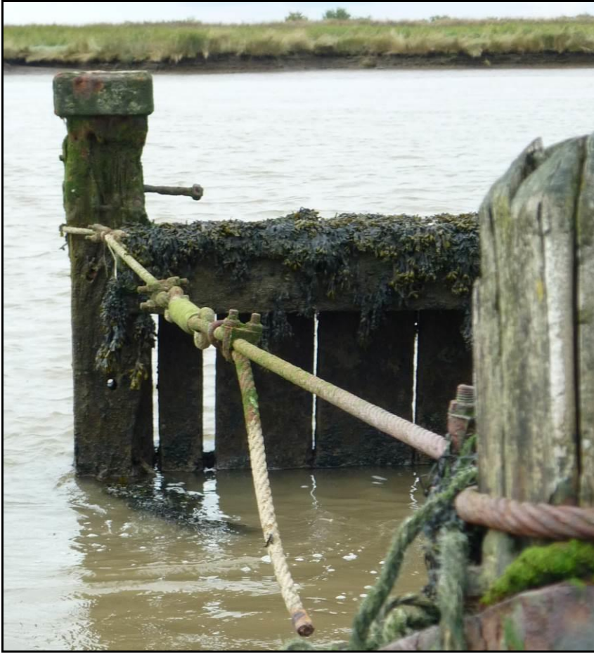
Photo: Steel wire tie (temporary strengthening)
