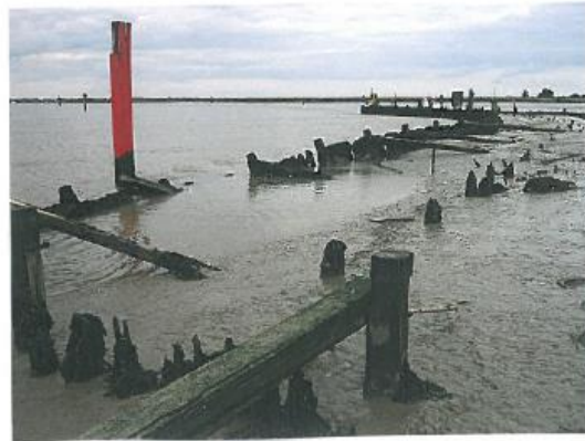
① FAILED PILING
