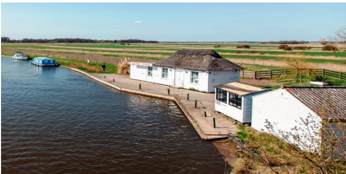
Photo: Acle Bridge site purchased by the BA
