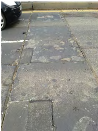
Typical view on Deck Board requiring probable replacement next financial year. d
