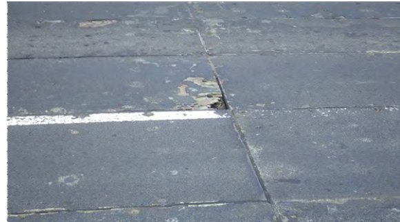
Broken Corner to Deck Board
