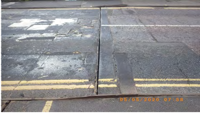
Steel Noising Bouncing Due to possible Broken Weld
