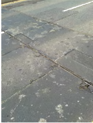
Typical view on Deck Board requiring probable replacement next financial year. a
