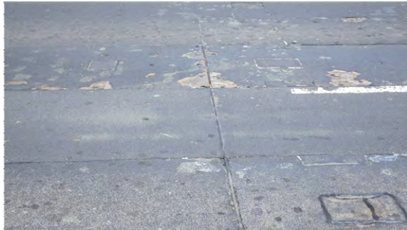
Typical Anti Slip Surface Lose
