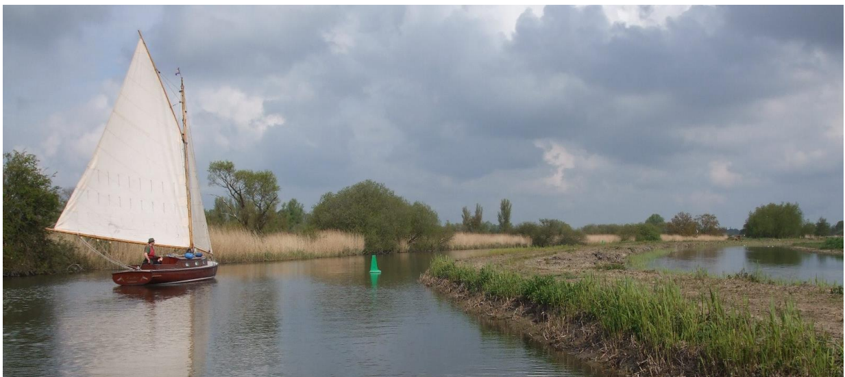
River Ant downstream of How Hill. Piling removed and old bank lowered as part of the Broadland Flood Alleviation Project. © Jeremy Halls
