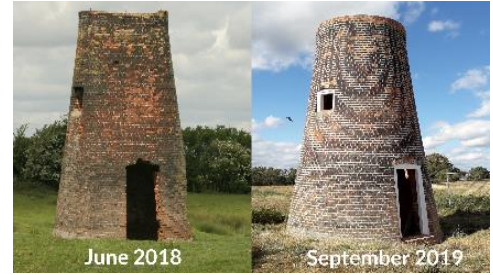
Photo: North Mill before and after restoration
