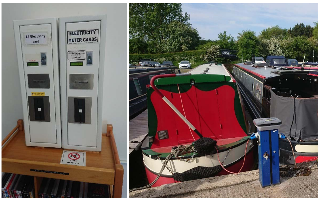
183 Electricity meter cards dispenser and electricity (and water) unit at Cowroast Marina.
