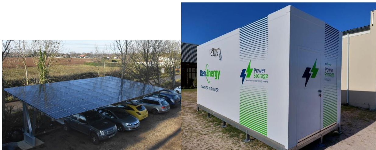
Figure A5.6: Solar canopy and static battery offering a renewable energy solution to ECP electricity supply.
