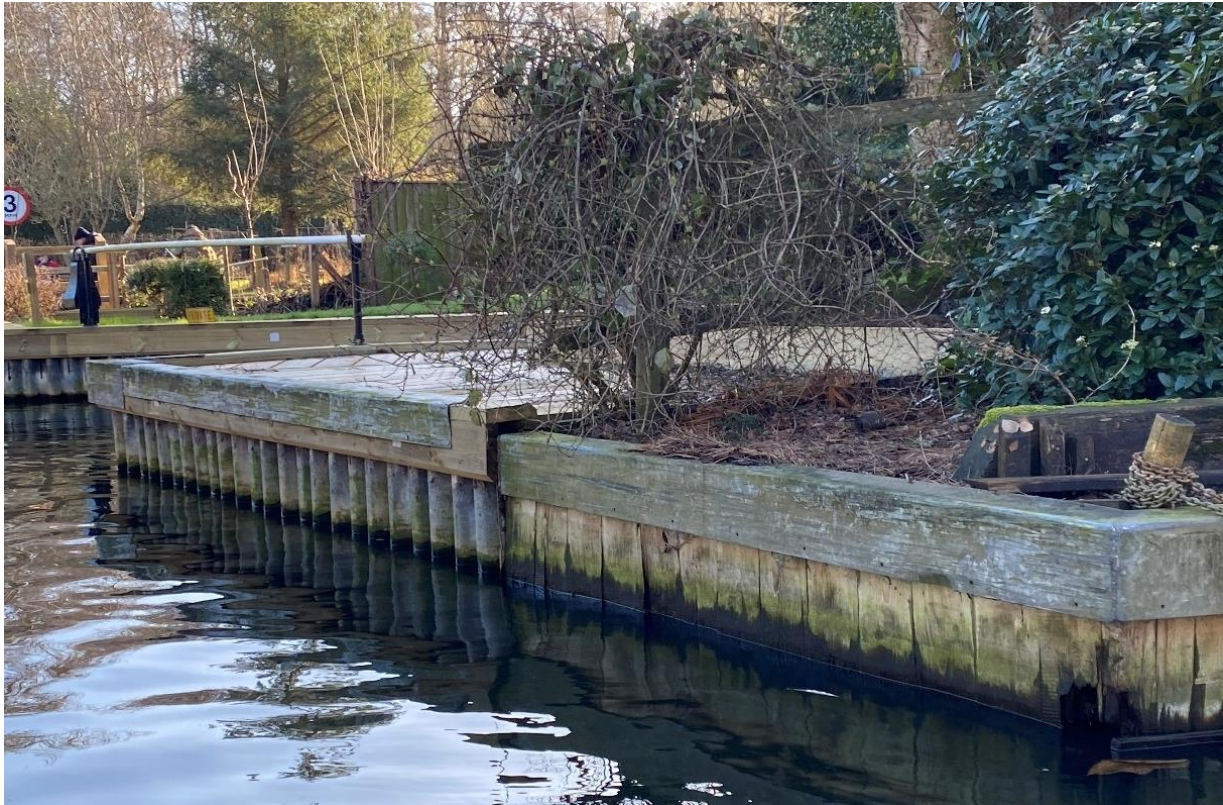
Above: Steel (left hand side) and timber (right hand side) quay heading, both with timber whaling boards and capping.
