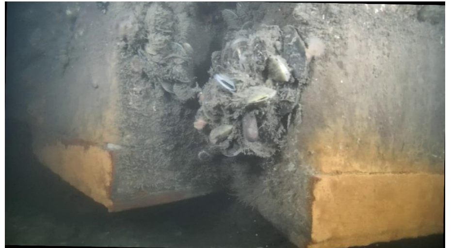
View of shoes on bottom of internal lock gates
