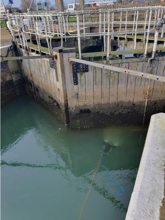
ROV preparing to descend along the lock gate
