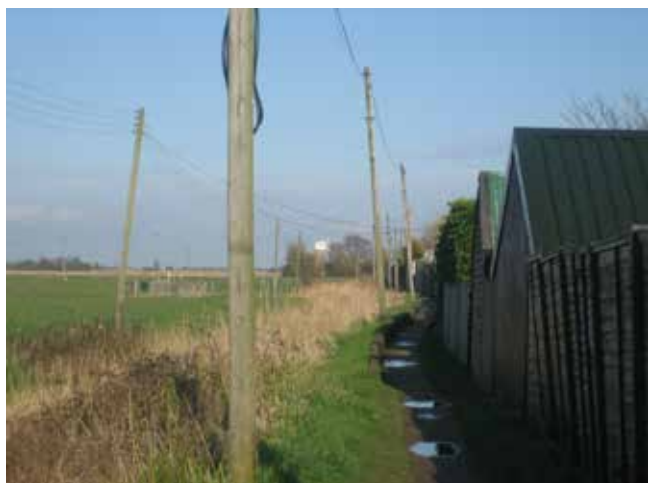
Phone and electricity poles and cables can create visual clutter. Lesley Marsden
