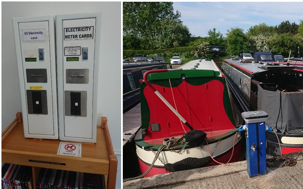
Electricity meter cards dispenser and electricity (and water) unit at Cowroast Marina.
