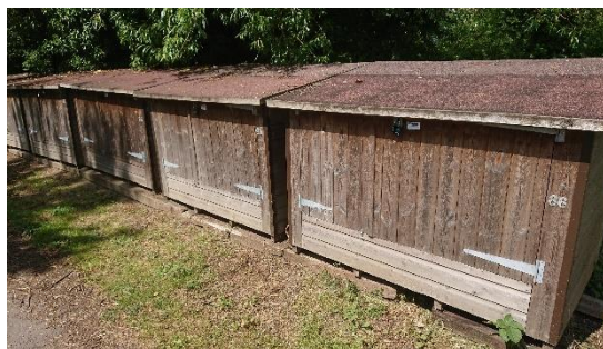
Storage lockers at Priory Marina
