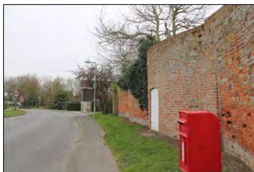
Figure 4 The Grade II listed serpentine wall.
