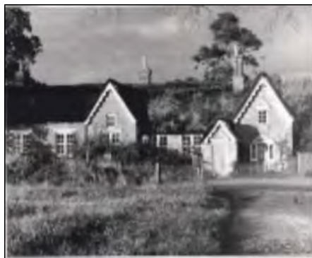
Figure 2 Worlingham Primary School
