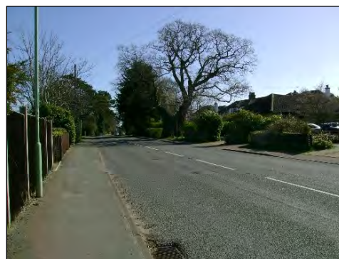
Figure 30. A third view looking east along the Lowestoft Road.
