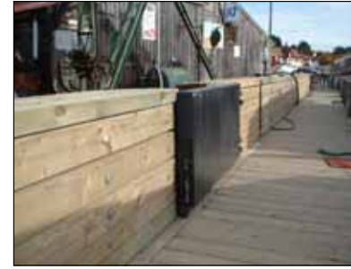
PHOTOGRAPH 1 SHOWING SIMILAR FLOODWALL CONSTRUCTED AT REEDHAM
