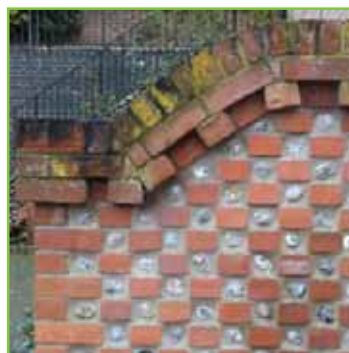
Red brick and flint cobble combined in a modern wall in Puddingmoor
