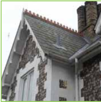
Painted brick and coursed, knapped flintwork in Puddingmoor, with decorative bargeboards, slates and chimney stack.
