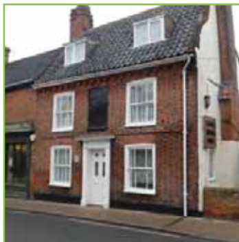
Burnt headers used in Flemish Bond brickwork combined with a blind central window, and decorative eaves detailing. A steep pantile roof with dormer windows
