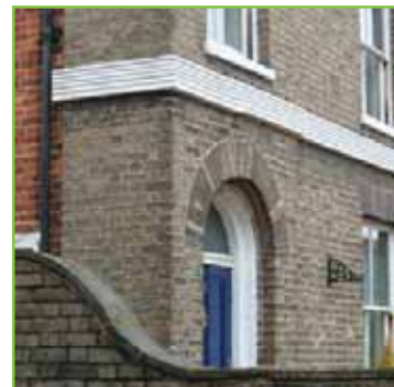
Gauged brick arches and a reeded string course in Station Road
